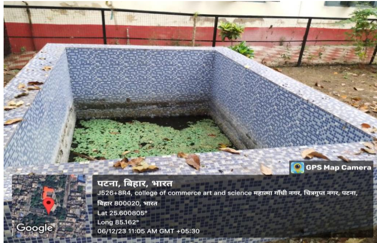
Fig.: Rainwater Harvesting unit installed near Zoology department.
